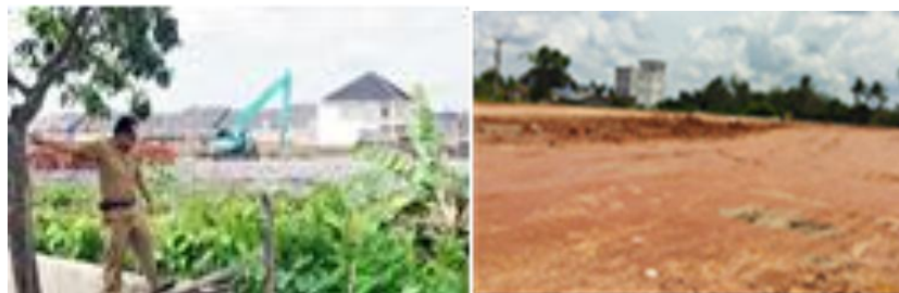
Figure 12. Swamp backfilling for housing development in Talang Jambe and Jakabaring.
